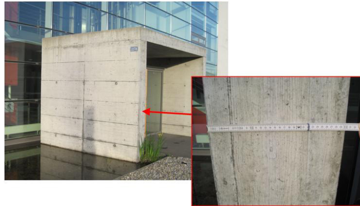
Figure 10: Concrete wall of 30 cm in thickness..
